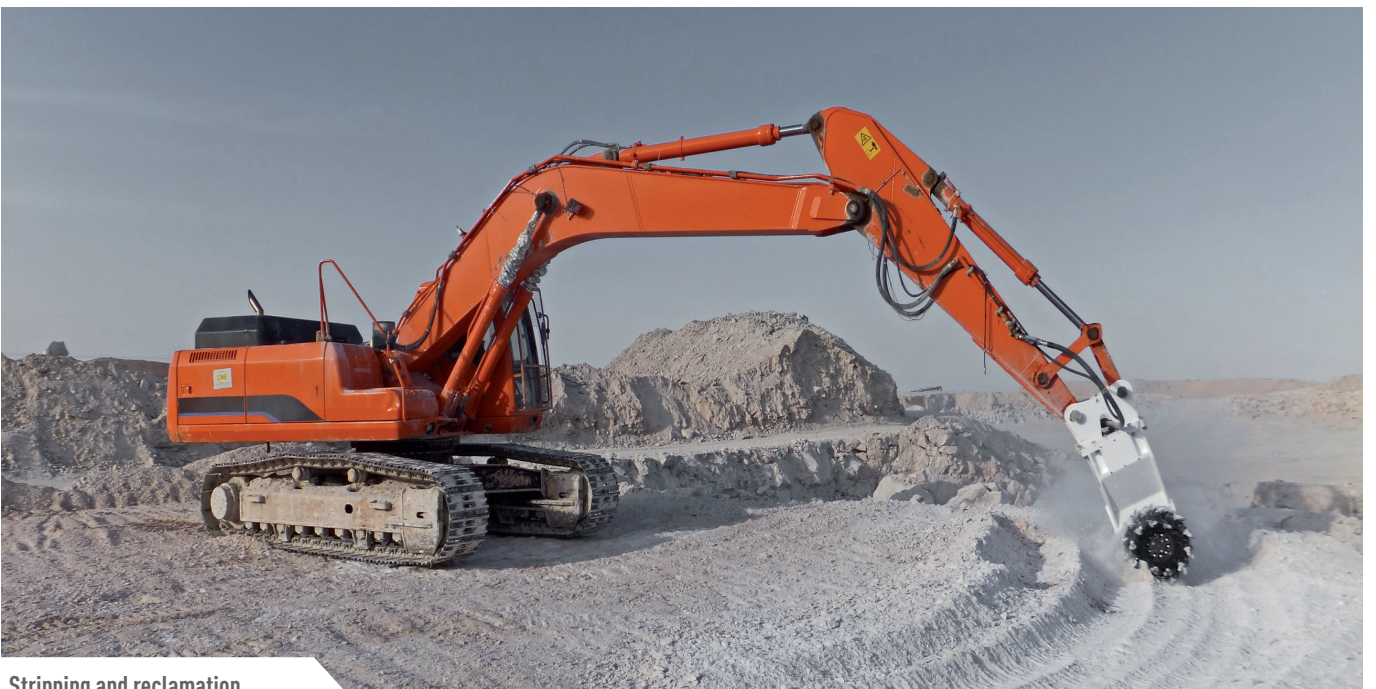
Stripping and reclamation
